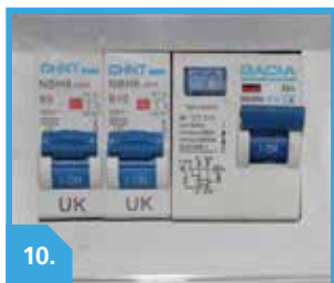
10. LOCATION OF CIRCUIT BREAKERS
