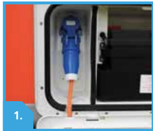
1. POWER SUPPLY TO OPUS
