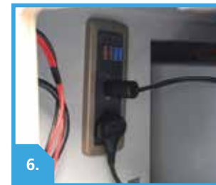
6. FUSE BOX LOCATION
