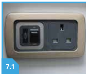
7.1 HEATER ISOLATION SWITCH
